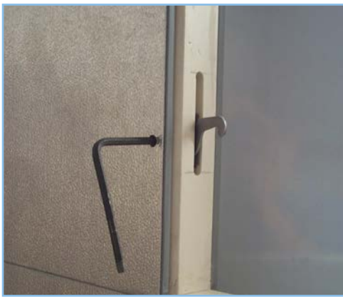
CAM-LOC FASTENING SHOWN WITH WRENCH
